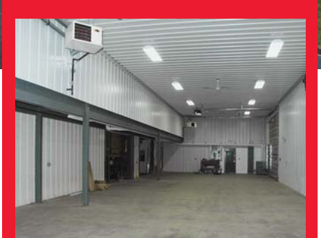
A view of the expanded warehouse prior to installation of cable handling and hydraulic pump servicing equipment.
