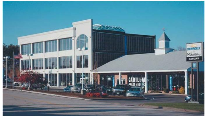
A view of the completed Phase II, showing temporary sidewall and existing showroom. Upon the completion of the move into the new showroom, the existing single-story showroom will be demolished, and the Phase III wing added to complete the project.
