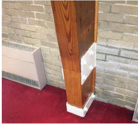
Above left: New steel plates were bolted on each side of the repair. Right: After repairs were made to the column.
